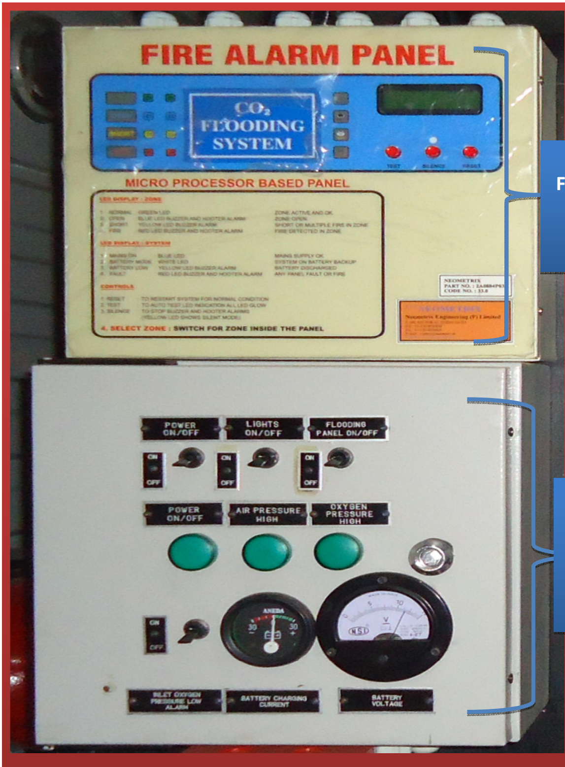
ELECTRICAL CONTROL PANEL & FIRE ALAM PANEL AS A WHOLE
